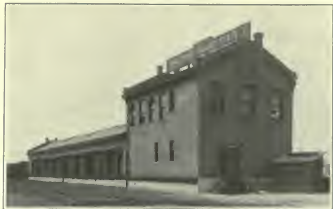
FIG. 322. FREIGHT HOUSES. Freight Station of the Chicago & Western Indiana Railroad, in the Englewood Yard at 66th Street, Chicago.
